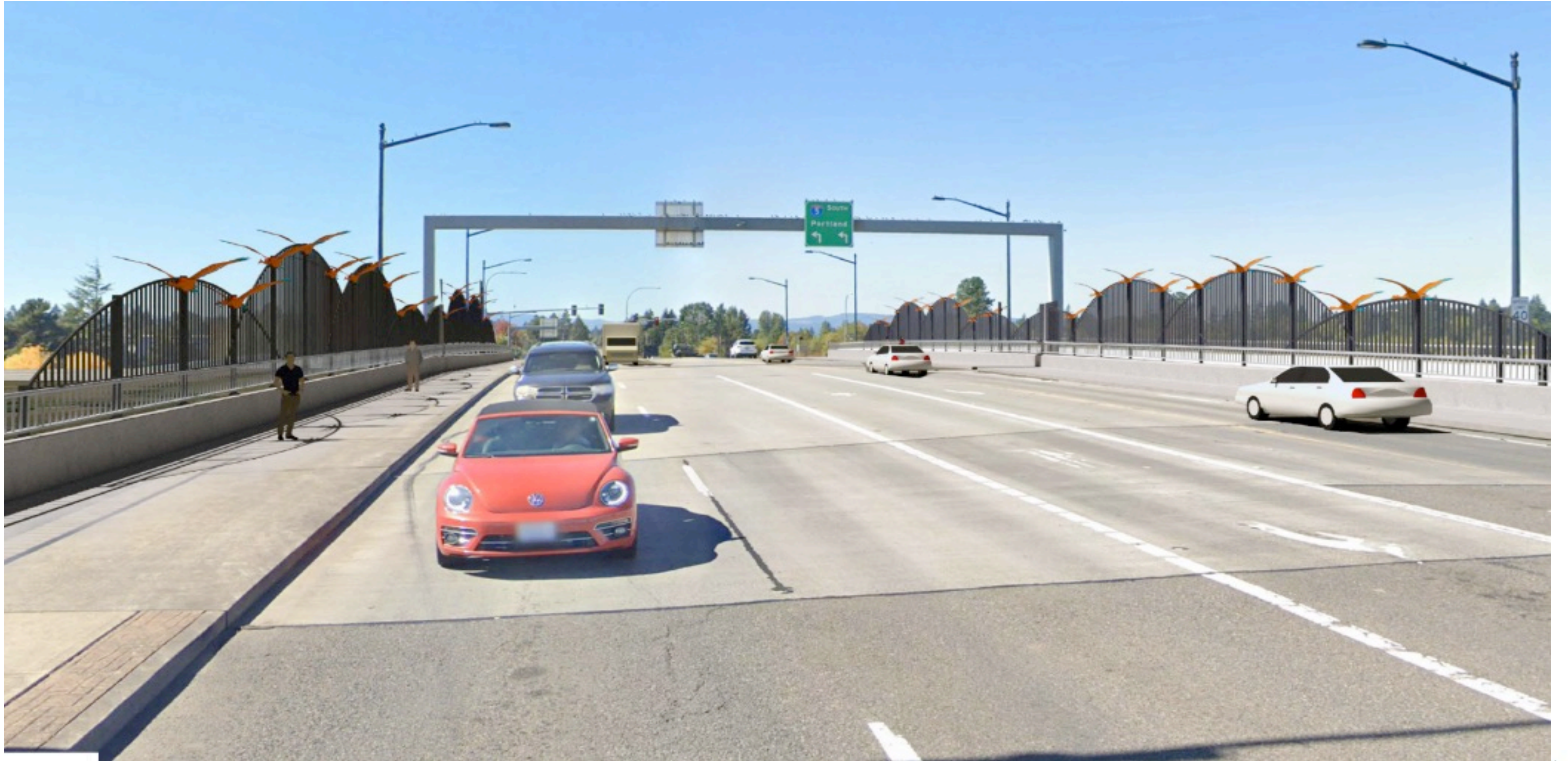
I-5 Pioneer Street Overpass
